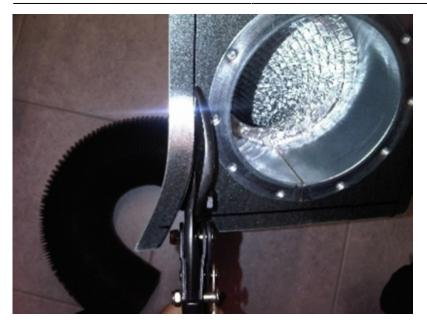
3. cut the front panel with tin snips 10cm opening for wall flange
